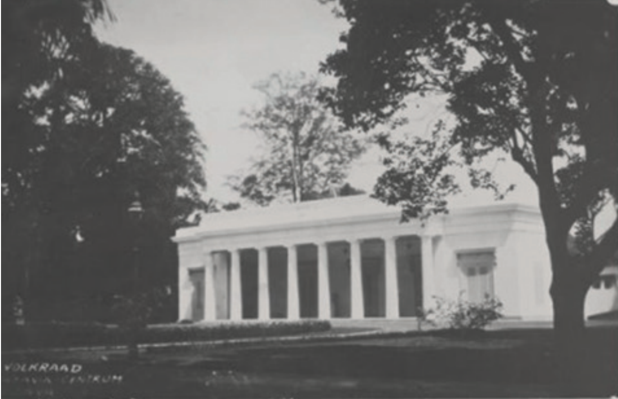
Volksraad Building in Batavia, c.1935.
